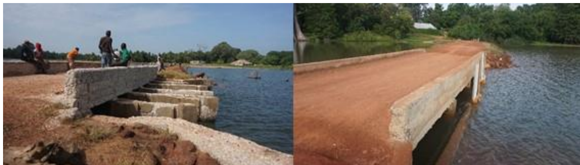
Figure 39 - Structures hydraulique de la vallée de Diacounda.
